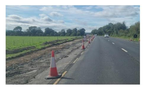
**Hazard:** There is concern that the surface of the greenway may fall within the barrier working width. Errant vehicles that impact with the VRS may deflect the barrier and impact with greenway users. Additionally, entrance and exit points to / from the greenway may be blocked by the VRS.
