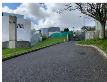
Image 12: Embankment between RCC and Letterkenny Tennis Club
