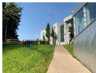
Image 13: Existing path along the front of RCC
