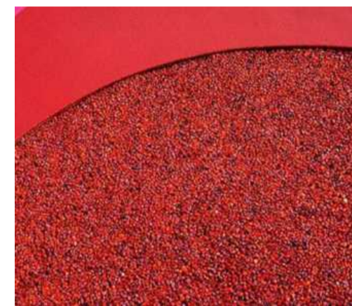
RED COLD COLOURED PLASTIC AND RED ASPHALT
