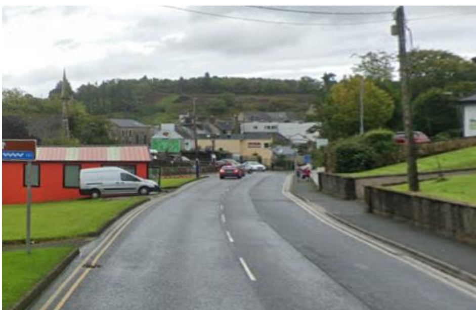
Figure 4-2 Existing Carriageway Width
