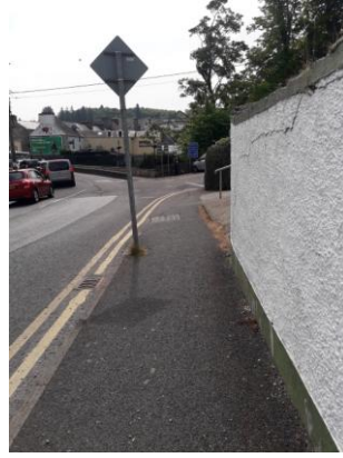
Plate 4. Looking east from southern side of road, towards bridge into Donegal Town (across River Eske).
