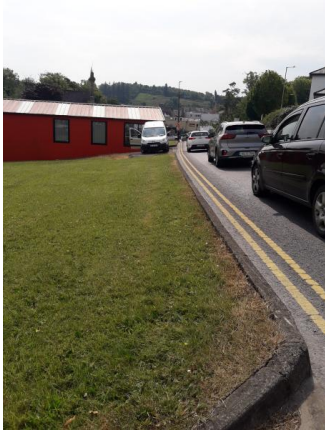
Plate 3. Looking east along proposed location for footpath.
