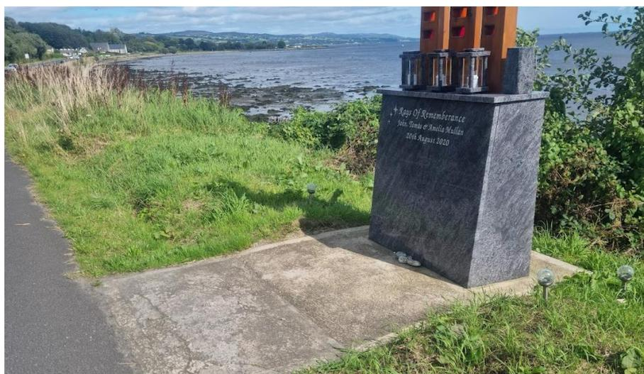
**Hazard:** Errant drivers may strike the monument resulting in vehicle occupant injuries. Additionally, the barrier will not achieve suitable restraint over the terminal length.
