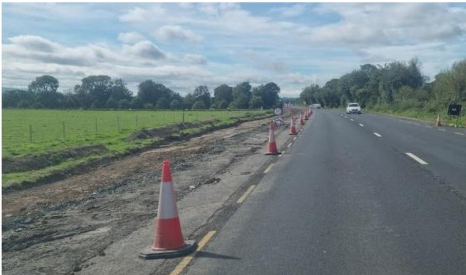
**Hazard:** There is concern that the surface of the greenway may fall within the barrier working width. Errant vehicles that impact with the VRS may deflect the barrier and impact with greenway users. Additionally, entrance and exit points to / from the greenway may be blocked by the VRS.
