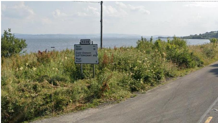
**Hazard:** Errant vehicle impact with the sign may result in vehicle occupant injury.
