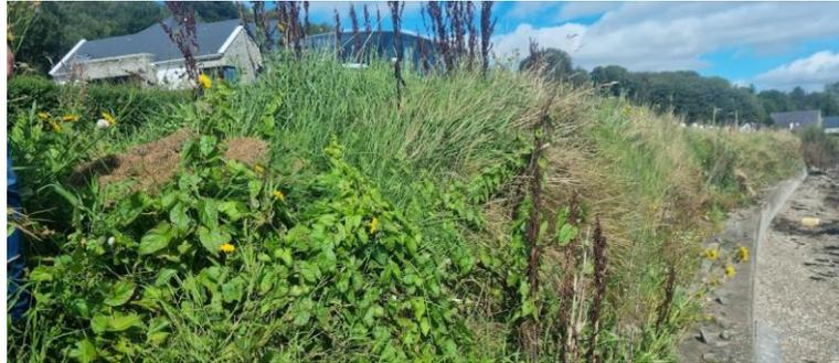
**Hazard:** There is concern that the ground to the rear of the barrier may fall away, particularly if the barrier is hit. The barrier may collapse and permit errant vehicles to enter the water hazard.
