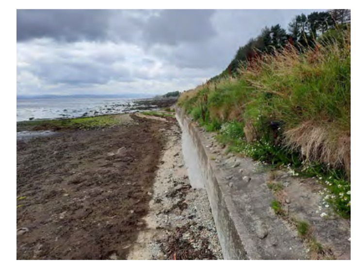
Existing concrete sea wall
