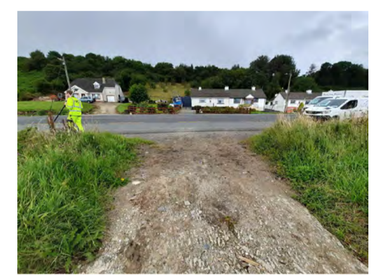
Existing shore access to be retained
