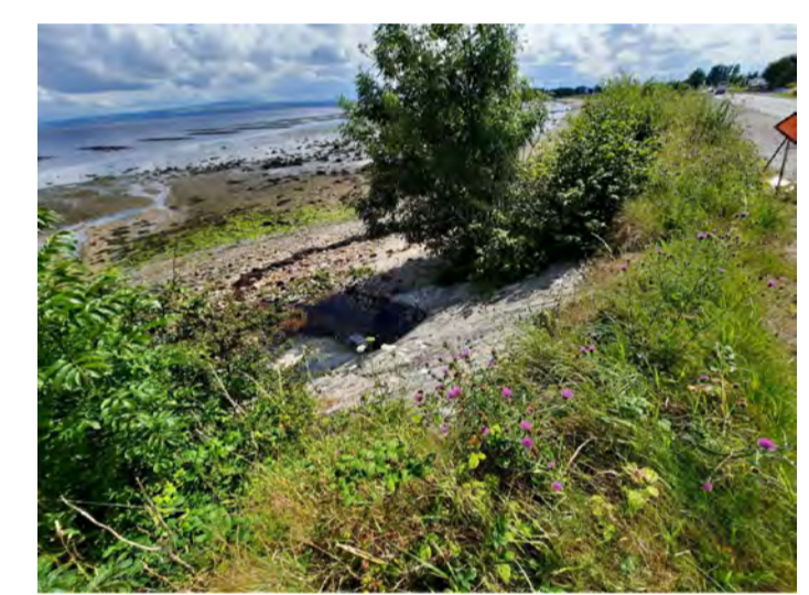
Existing drain outlet
