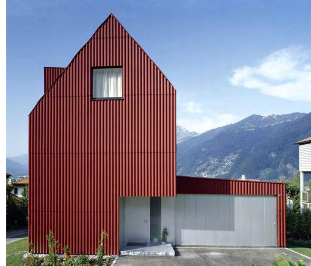
2. Corrugated Fibre Cement Panels *Current external render images are shown with this material*
