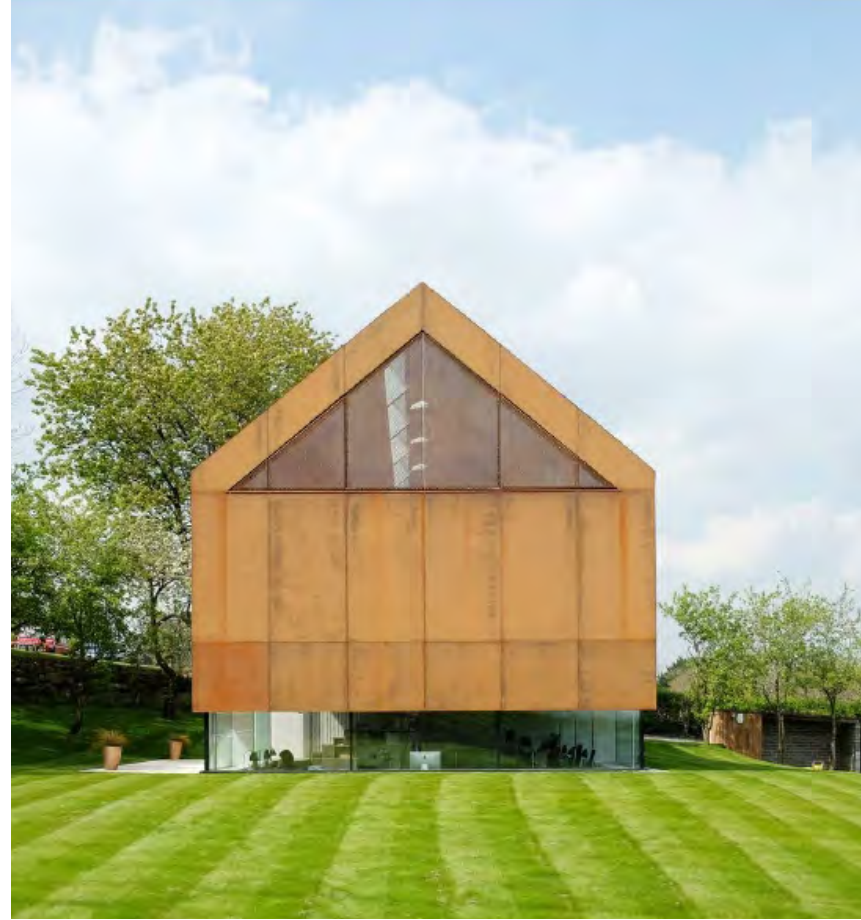
1. Corten Steel Cladding
