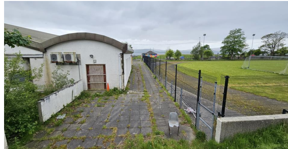
Plate 4: Northern boundary of Leisure Centre showing paved area.
