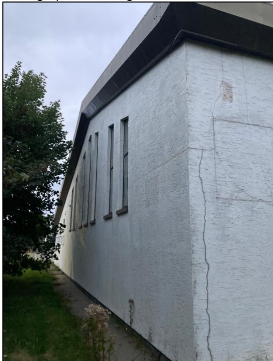
Photograph 2 Existing leisure centre
