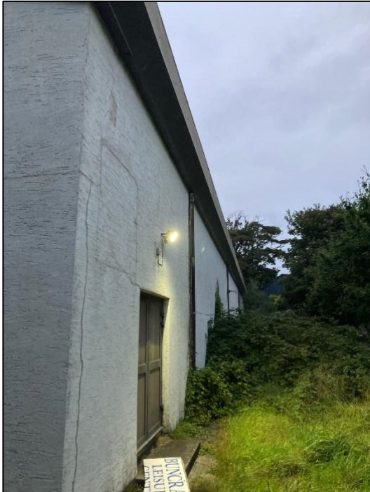
Photograph 1 Existing leisure centre
