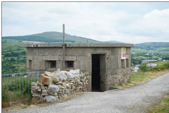
Plate 3.19: Blockhouses – solid concrete structures with flat roofs [June 2022]
