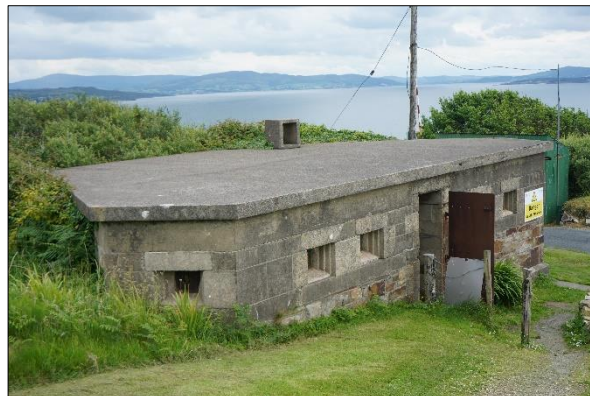
Plate 3.20: Blockhouses – solid concrete structures with flat roofs [June 2022]
