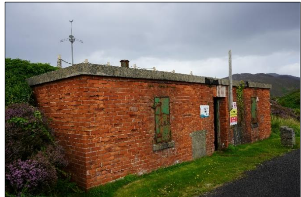
Plate 2.46: PRA – all other small structures and shelters were assessed as being of negligible suitability for roosting [August 2023]
