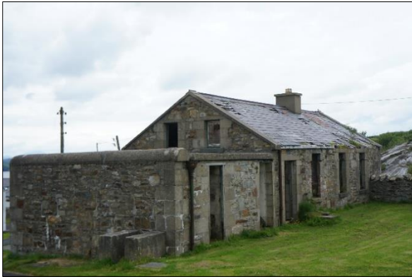
Plate 2.40: PRA – derelict stone/brick structures with slate/tile roofs were assessed as being of low suitability for roosting [June 2022]
