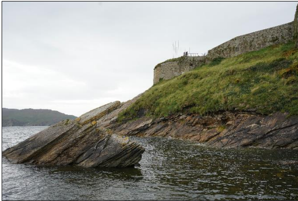
Plate 3.5: Lower Fort – Lough Swilly Walkway to be constructed on the seaward side of the fort [August 2023]
