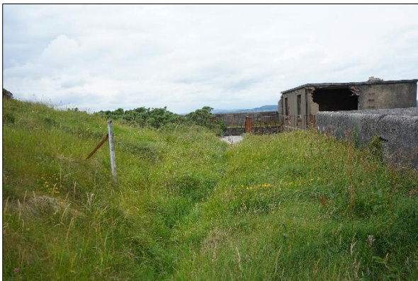
Plate 3.2: High Fort / Redoubt – discontinuous & degraded heathland/grassland will be lost from the interior [June 2022]
