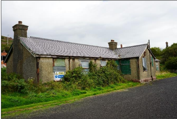
Plate 3.17: Brick Buildings – 1 of 2 adjacent buildings to be restored and repurposed as Welcome Buildings [August 2023]
