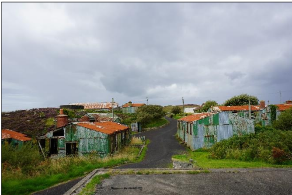
Plate 2.16: BL3 Buildings & Artificial Surfaces, ED2 Bare Ground, GA2 Amenity Grassland, overgrown BC2 Horticultural [August 2023]
