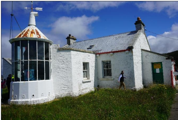
Plate 3.9: Lighthouse – current condition & presentation of the buildings and curtilage [July 2022]
