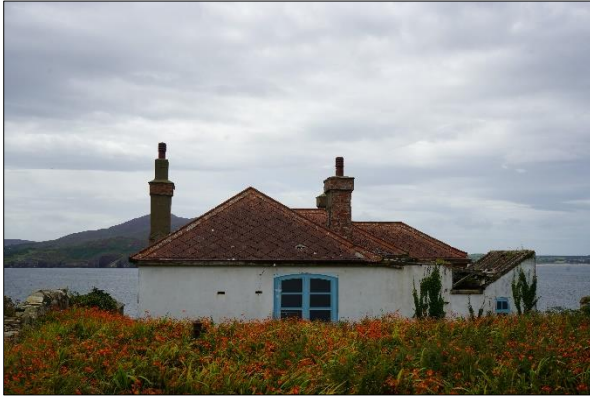
Plate 2.23: Montbretia Crocoshmia × crocoshmiiflora – dense stands surround the derelict/disused buildings [August 2023]
