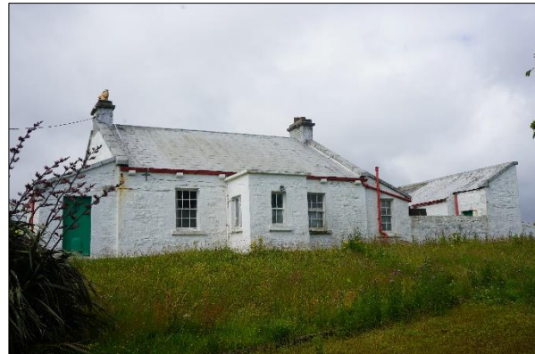
Plate 3.10: Lighthouse – current condition & presentation of the buildings and curtilage [July 2022]
