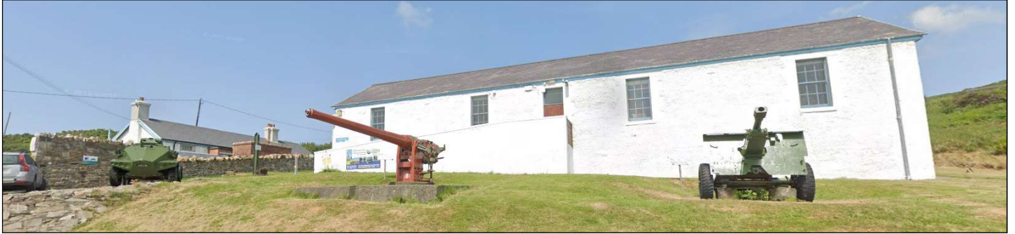
Plate 14: View of barracks 'A' Block from the car park at Fort Dunree Road facing east
