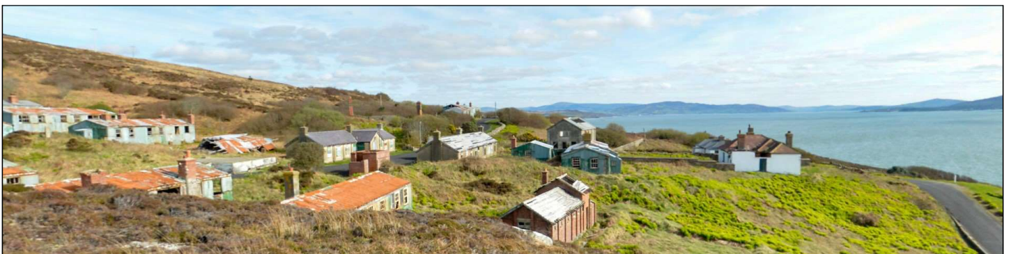
Plate 17: The front row of building (right to left) is the Bath House, Hut 6 and Hut 5. The back row of building (right to left) is the N.O. Quarters, the Sergeants Mess, barracks 'D' and 'C', Huts 7, 8 and 9 facing south
