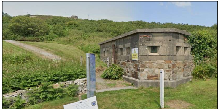
Plate 8: View of a stone sentry building located to the north side of Fort Dunree Road facing north west
