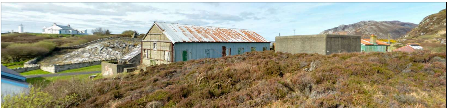
Plate 16: View (left to right) of Dunree Lighthouse and Lighthouse Keeper's House, the drill shed and a storage tank facing north
