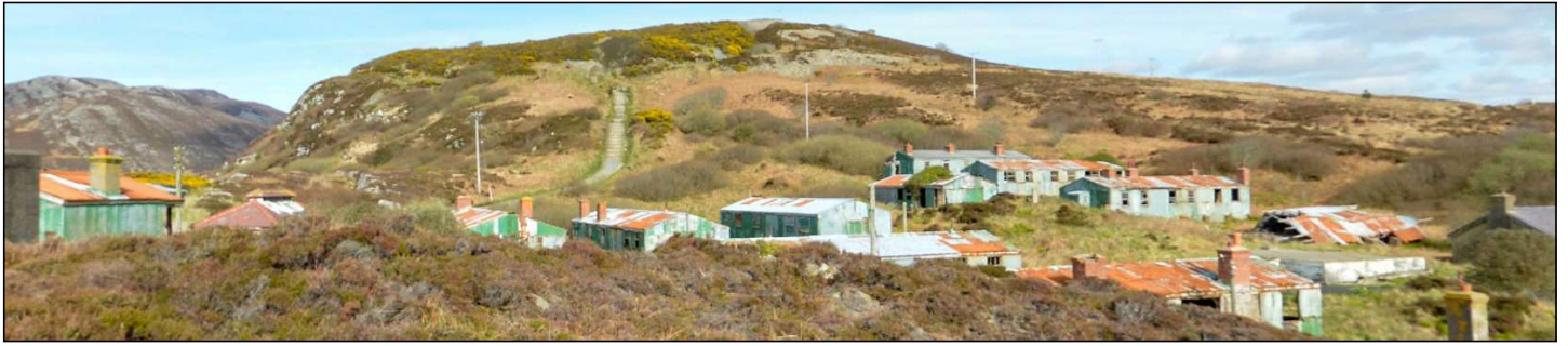
Plate 17: View across from the Ordnance Ground towards Dunree Hill and the battery located at the summit facing east
