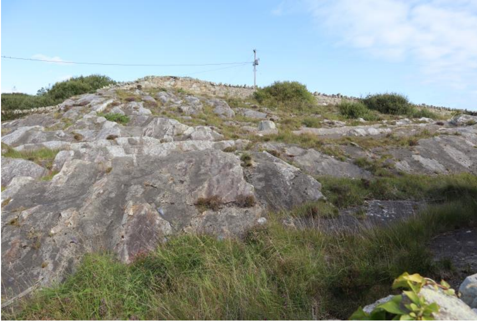
Figure 123 – 27.04 Water Catchment Area
