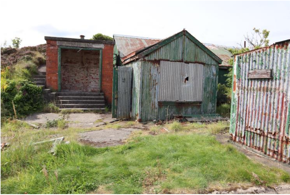
Figure 101 – 17.02 Oil storage shed
