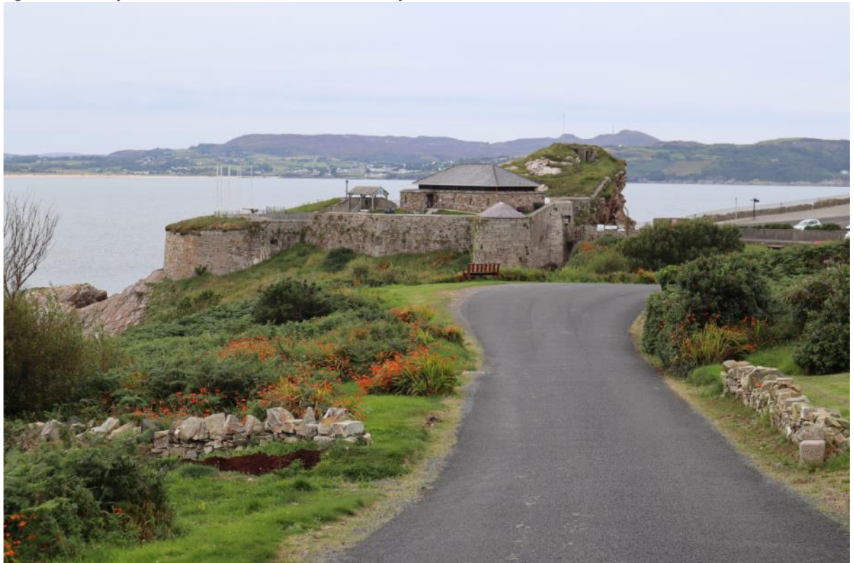
Figure 5 – view of Dunree Fort from south; hipped roof structure & shelter are modern additions affecting the character and visual interpretation of the gun-emplacement; otherwise, structures are substantially as reconstructed and re-armed circa 1895
