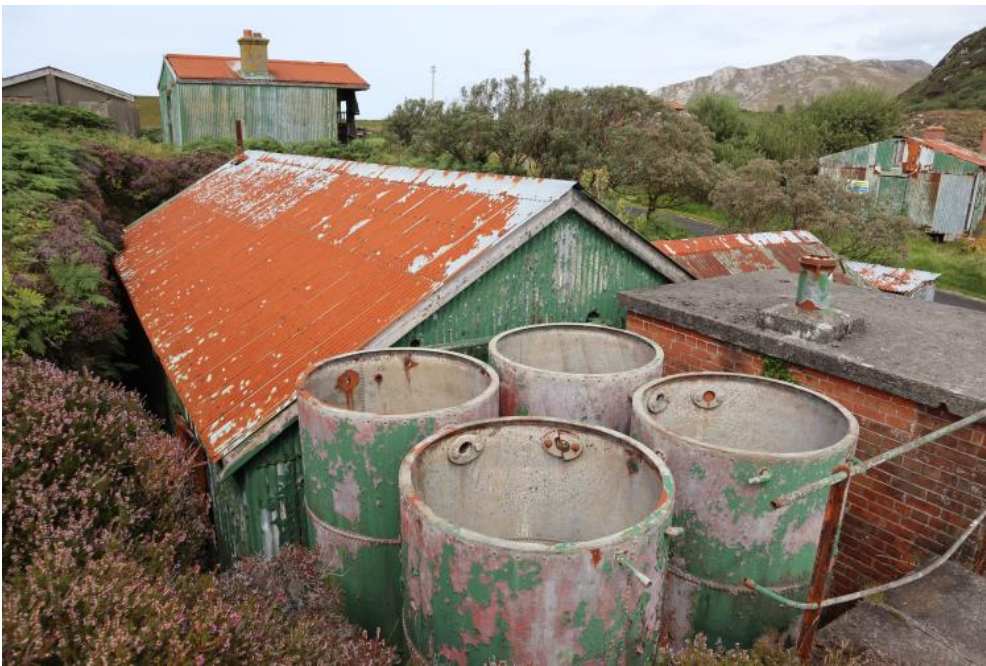
Figure 102 – 17.03 Oil fuel, Cistern & Cooling Tanks
