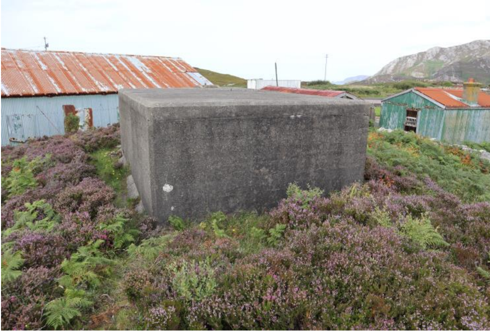
Figure 103 - 17.04 8,000 Gallon Tank & water supply network
