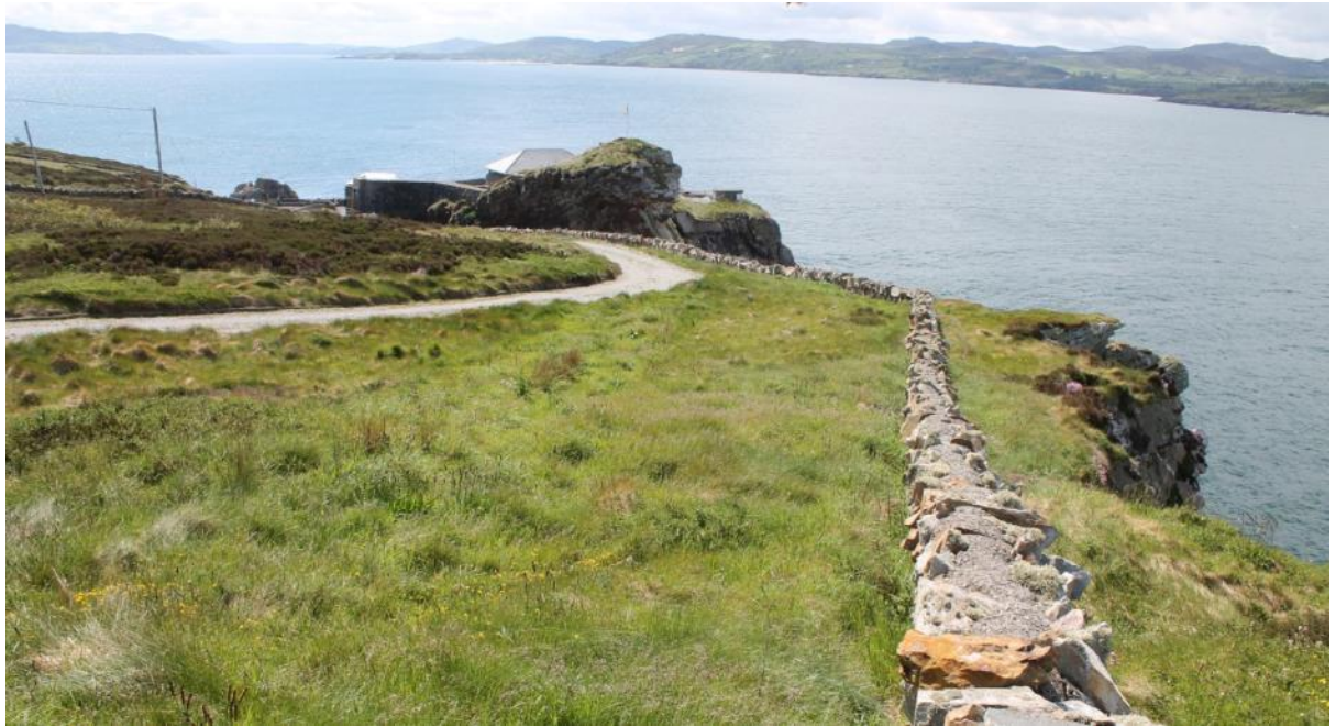
Figure 8 – view of Dunree Fort from the lighthouse grounds to the north
