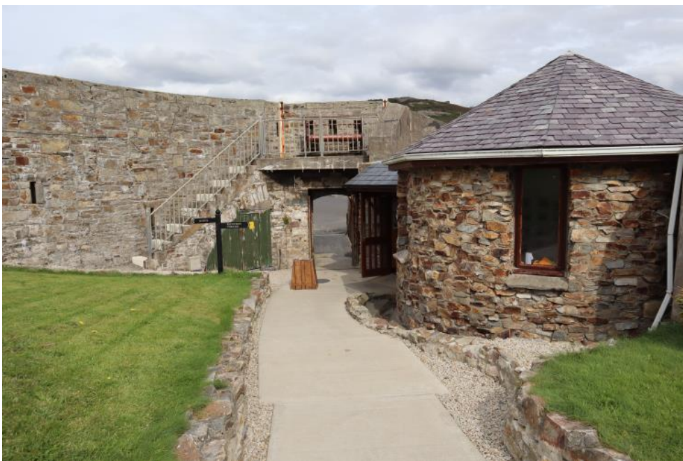
Figure 130 – 31.3 Sales Office (former fuel storage)
