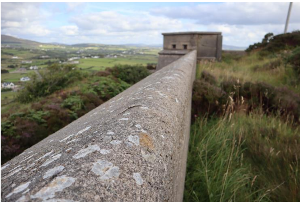
Figure 54 - 3.00 Redoubt Fort - Scarp Wall
