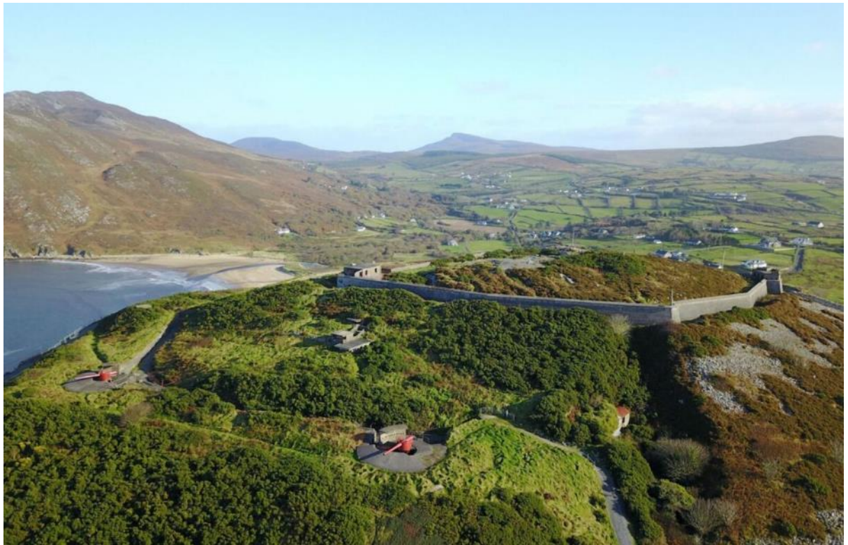
Figure 17 – elevated view of hill battery & redoubt fort; the structure largely unchanged since circa 1900 Image: © Donegal Daily
