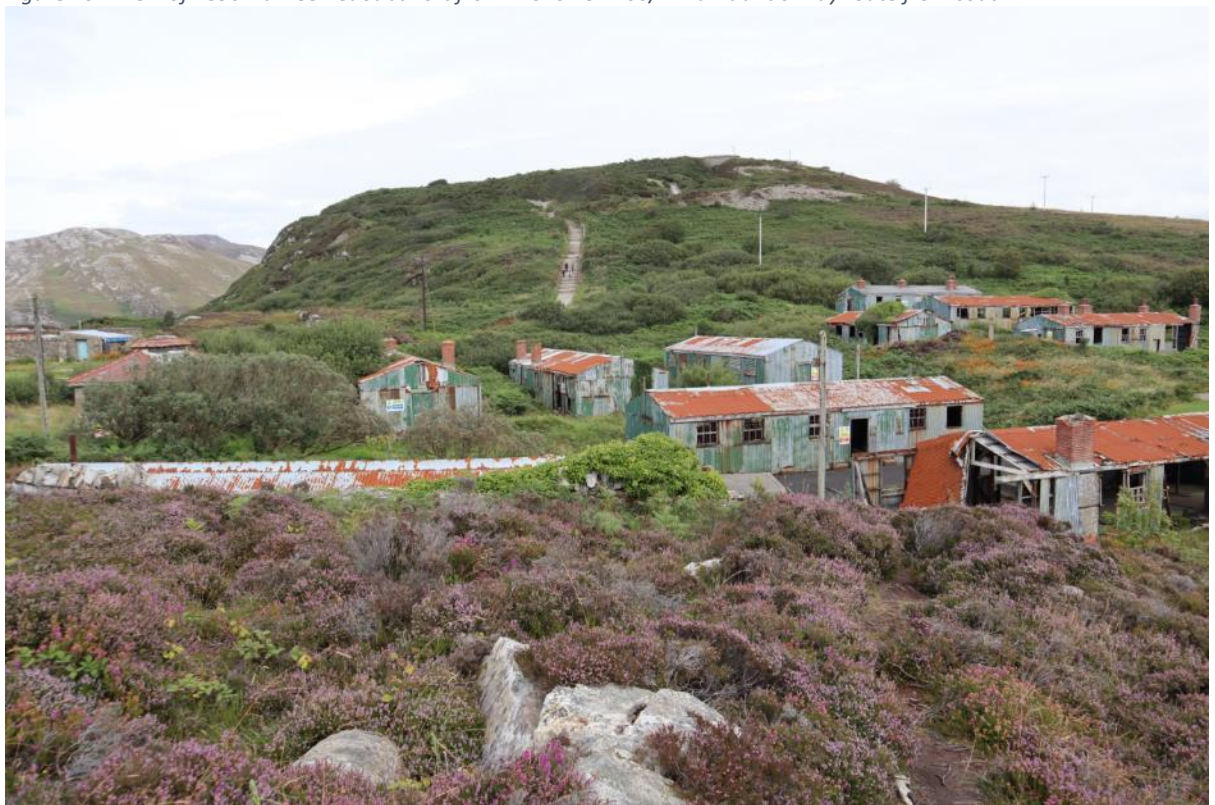
Figure 11 – view of 'hutment' towards Dunree Hill & Redoubt Fort; the iron clad timber hutment on the former camping grounds expanded mostly circa 1902 to 1912 to serve the expanded artillery base & further reinforcement during WW1
