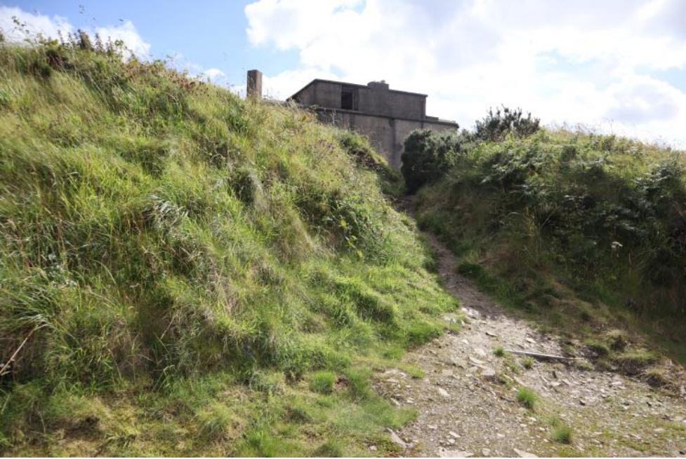
Figure 55 - 3.01 Guardhouse or Caretaker's Quarters
