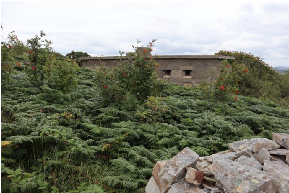
Figure 50 - 2.03 Block House 'C'
