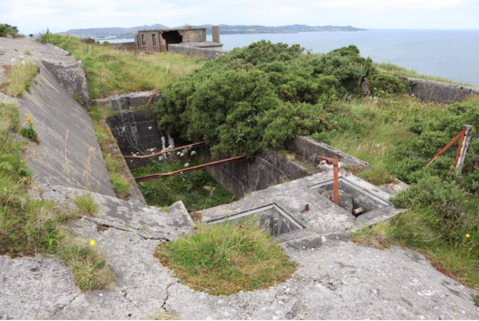
Figure 61 - 3.05 Water Storage/ Collection Tank
