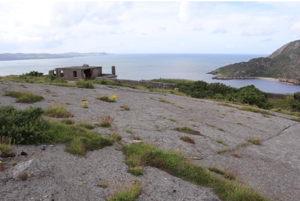
Figure 62 - 3.06 Rainwater Collection/ Catchment Area
