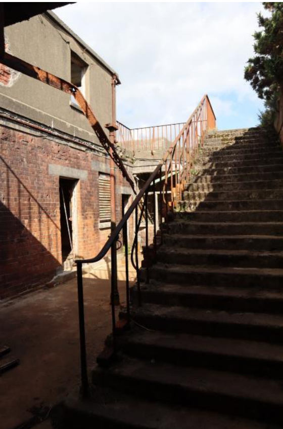
Figure 56 - 3.01 Guardhouse or Caretaker's Quarters
