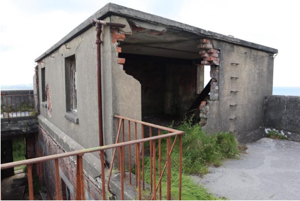
Figure 57 - 3.01 Guardhouse or Caretaker's Quarters
