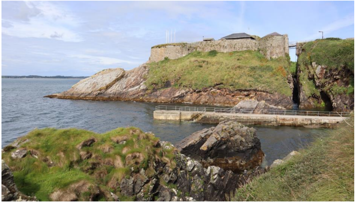
Figure 6 – view of Dunree Fort from south; large masonry bastions and revetments are as constructed circa 1810
