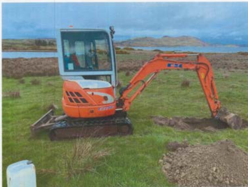
Trial Hole being Excavated
