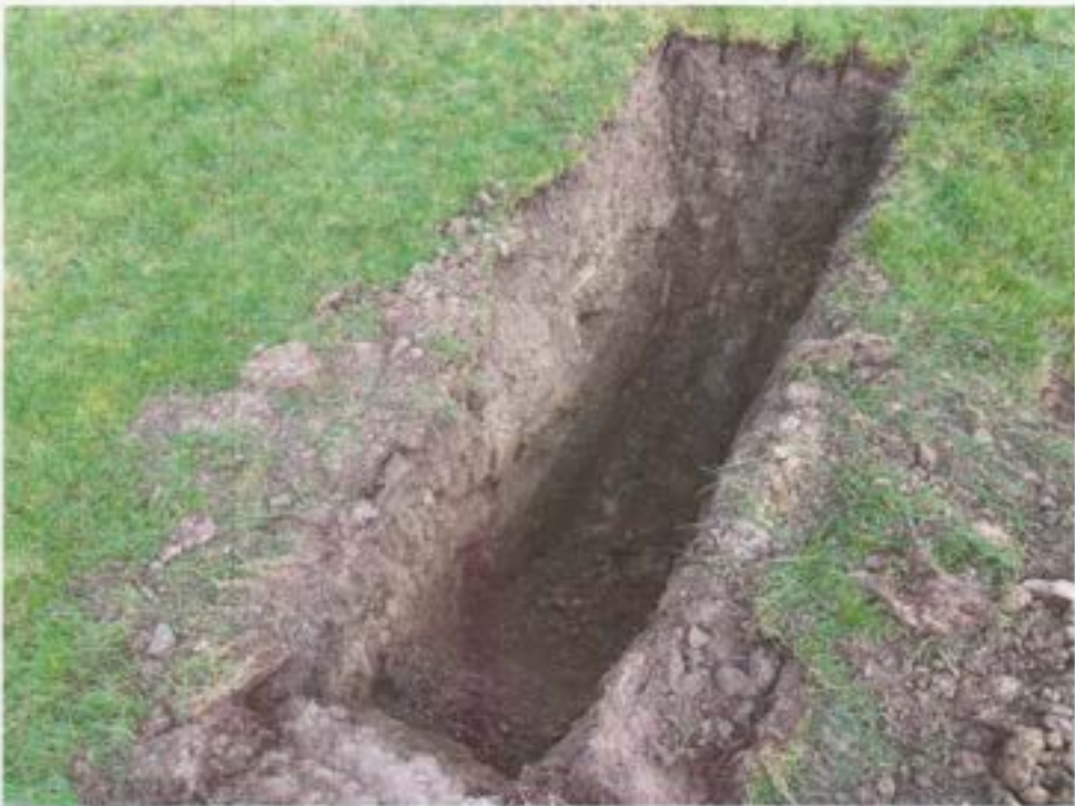
Trial Hole after Excavation
