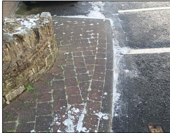
Figure 2-1 Constrained footpath width at existing/proposed raised crossing point
