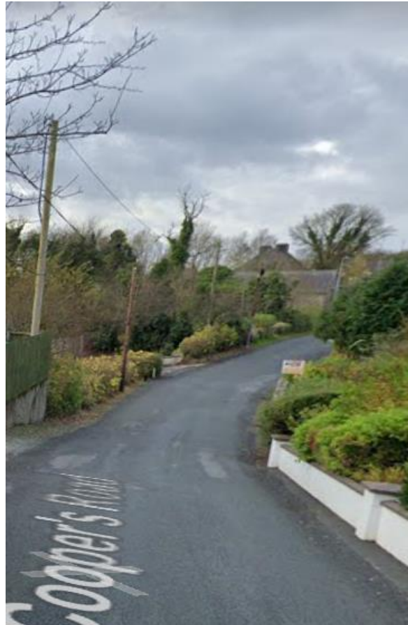
Figure 4-5 Lack of Footpath Provision
