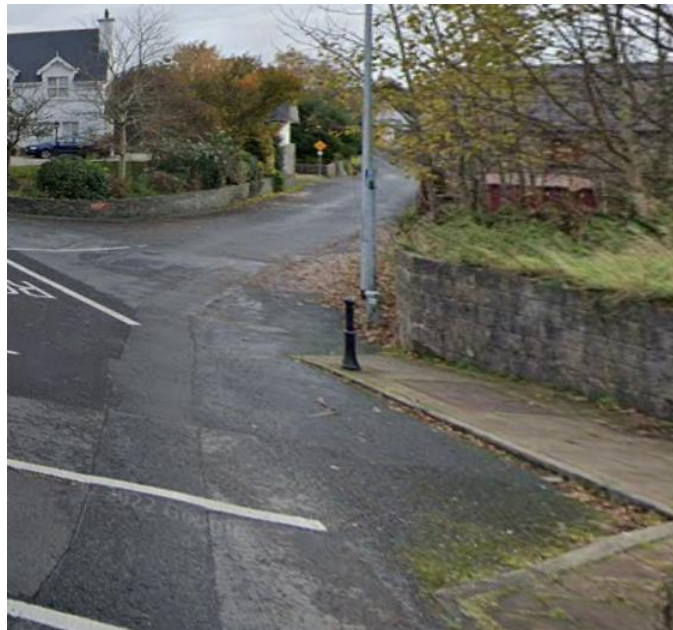
Figure 4-3 Existing Footpath at Market Square
