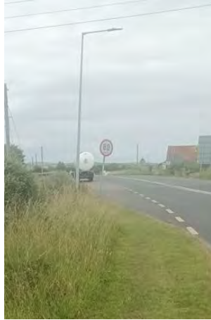
Plate 2-1: Existing Lighting Column
