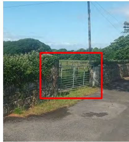
Plate 2-14: Existing Access (Chainage 3400m)
