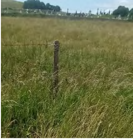
Plate 2-15: Existing Concrete Posts
