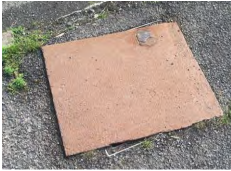
Plate 3-5: Existing Access Chamber
