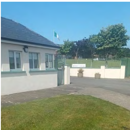
Plate 2-21: Existing Pedestrian Access
