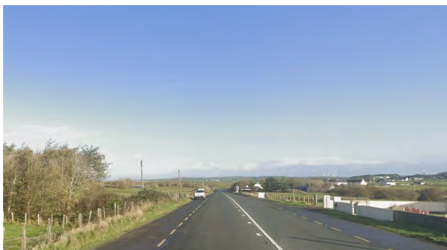
Figure 4-1 Existing Carriageway Width
