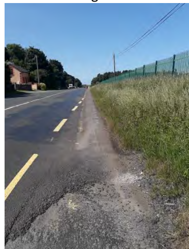
Plate 6. Looking west along Finner Camp, hard shoulder narrows, surface water percolates to ground.
