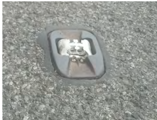
Plate 2-10: Existing Studs
