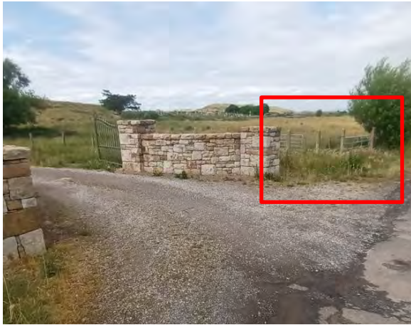
Plate 2-11: Existing Access (Chainage 275m)
