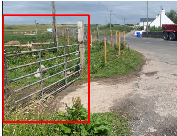
Plate 2-12: Existing Access (Chainage 525m)
