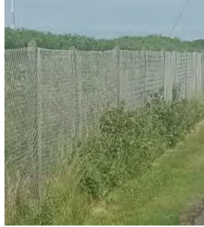
Plate 2-16: Existing Concrete Posts
