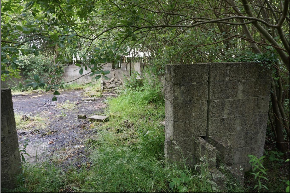
Photograph 4.1: Partially constructed buildings on site.
