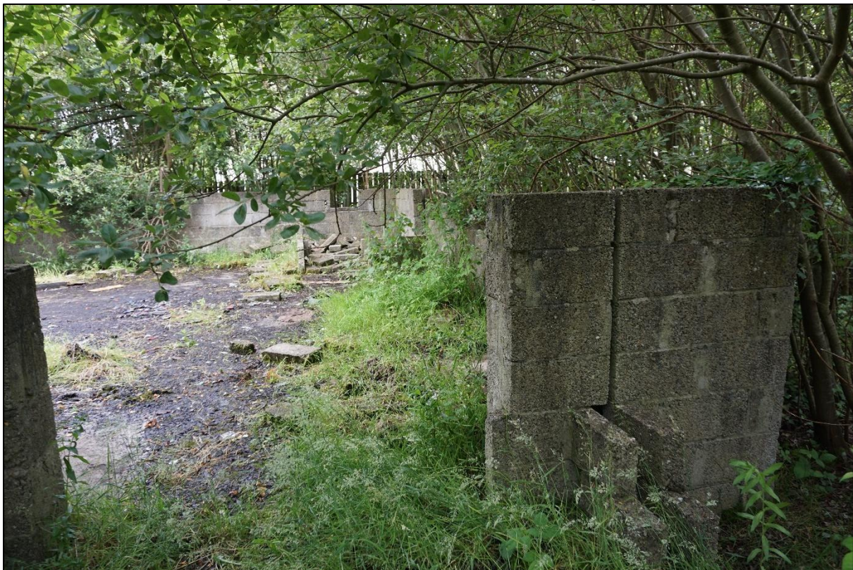
Photograph 4.1: Partially constructed buildings on site.
