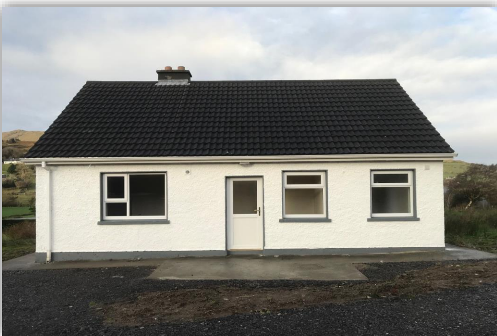
Cashel Ardara Dwelling Refurbishment - After
