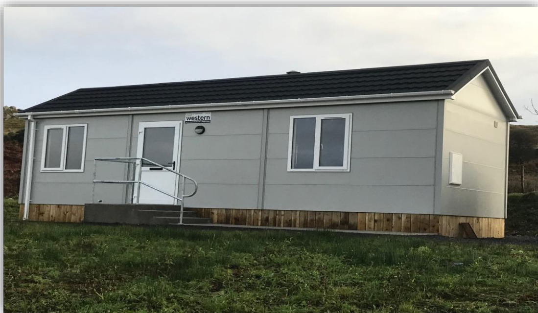
Cashel Ardara Single Unit accommodation replacement – After
