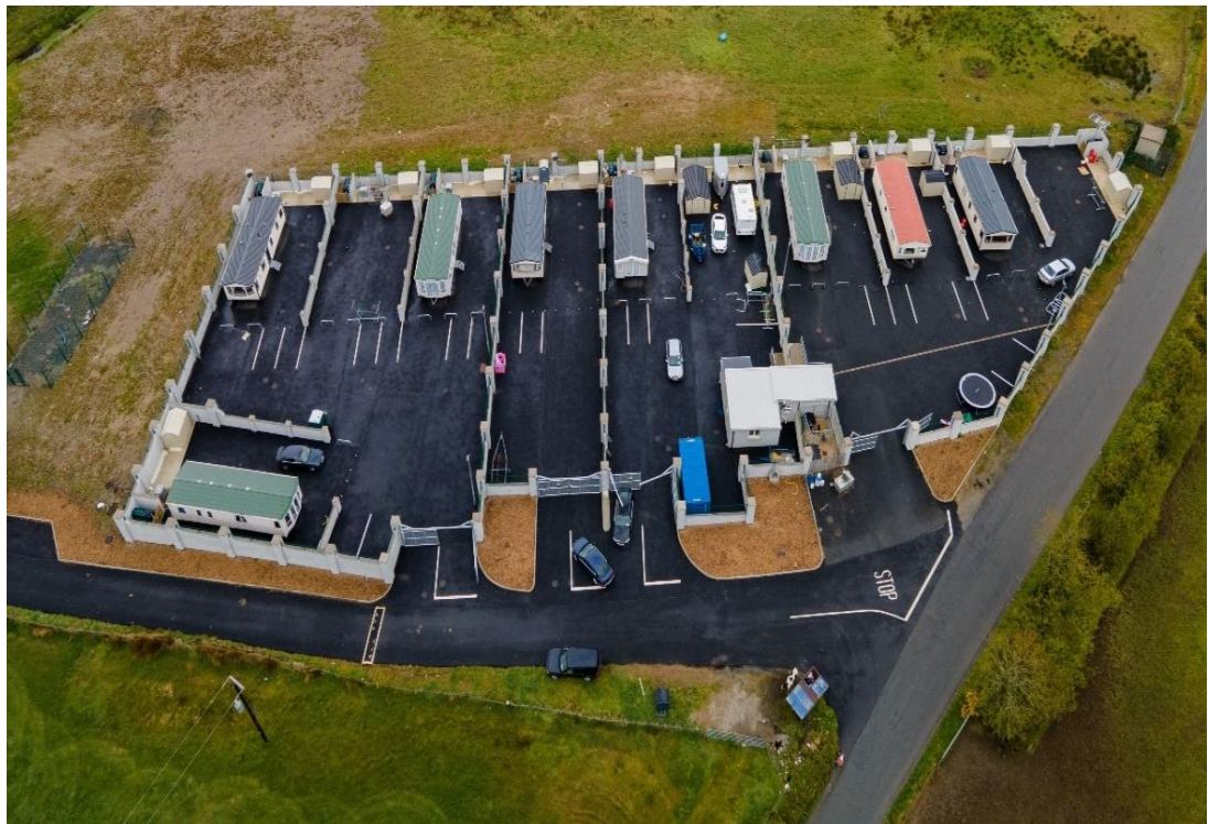
Big Isle halting site – Refurbishment & Extension
