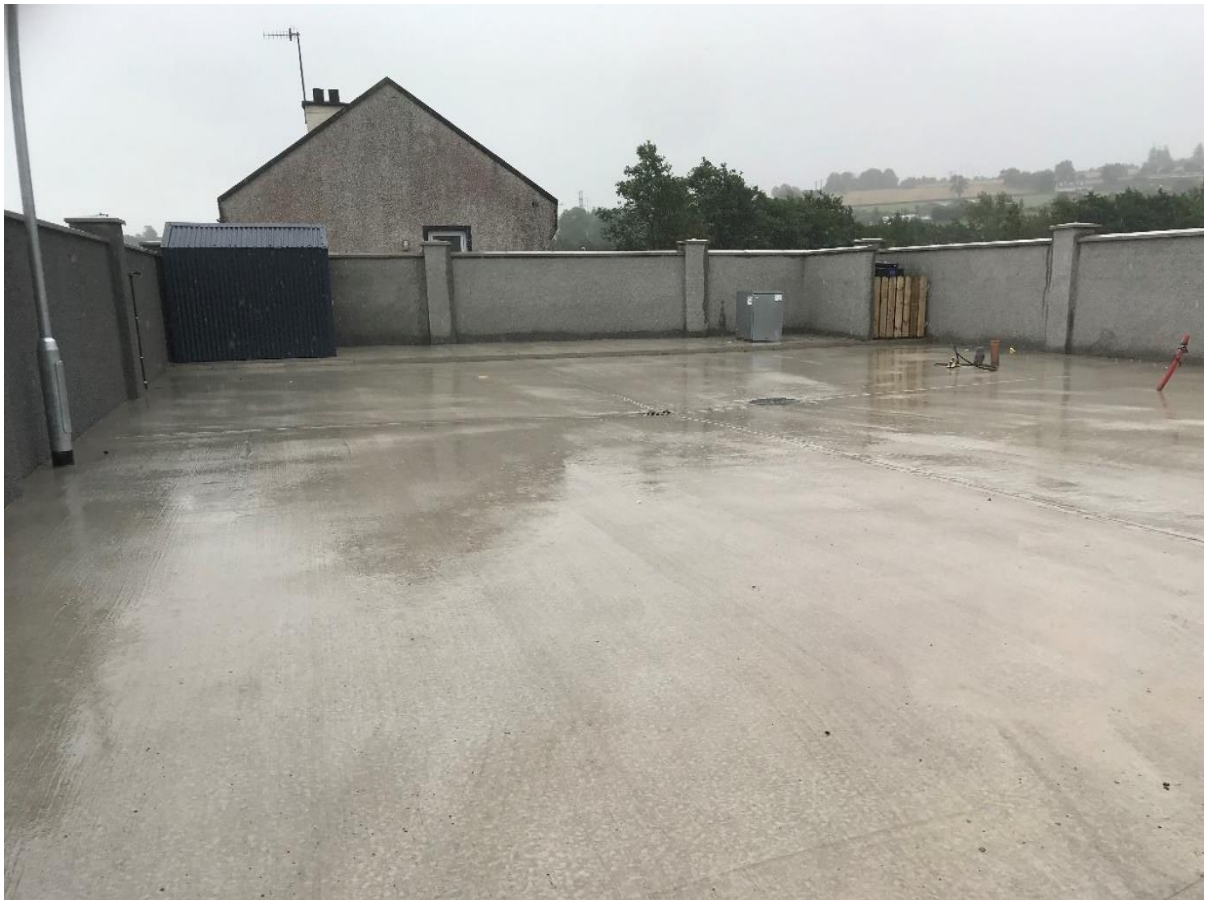
Canal Road Permanent Bays Construction - After
