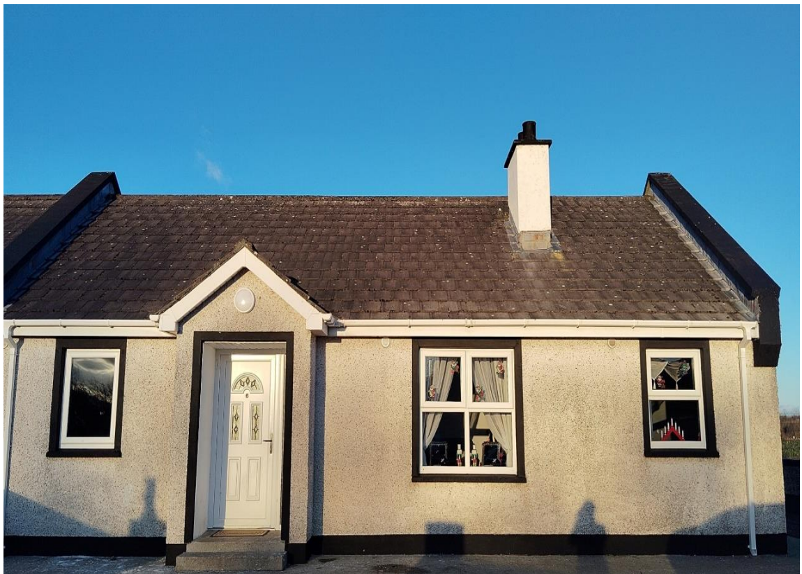
Canal Road Group Housing Dwelling Refurbishment
