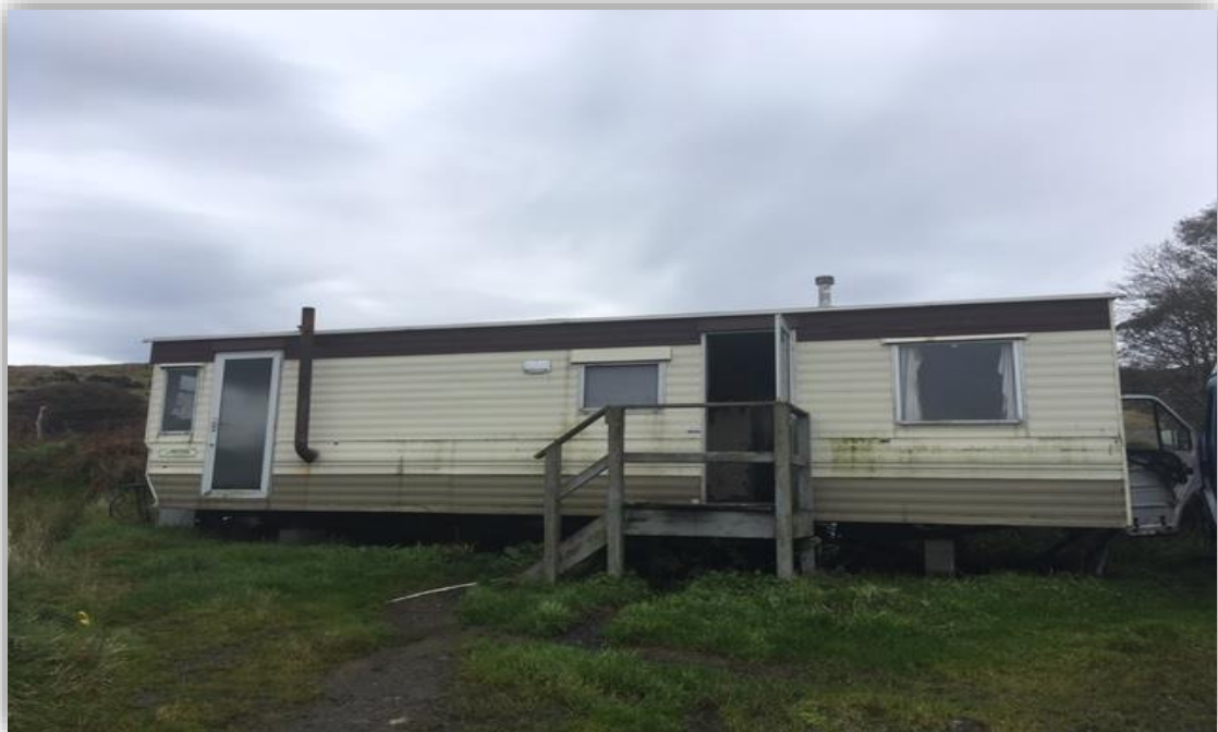
Cashel Ardara Single Unit accommodation replacement - Before
