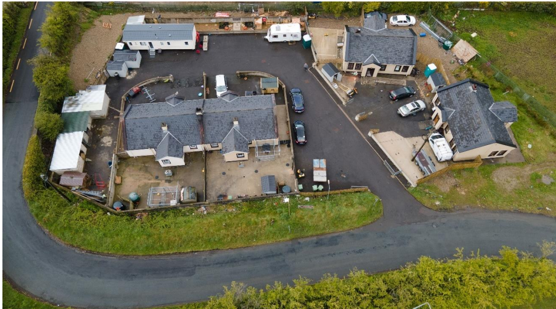
Cullion Road Group Housing scheme, Letterkenny
