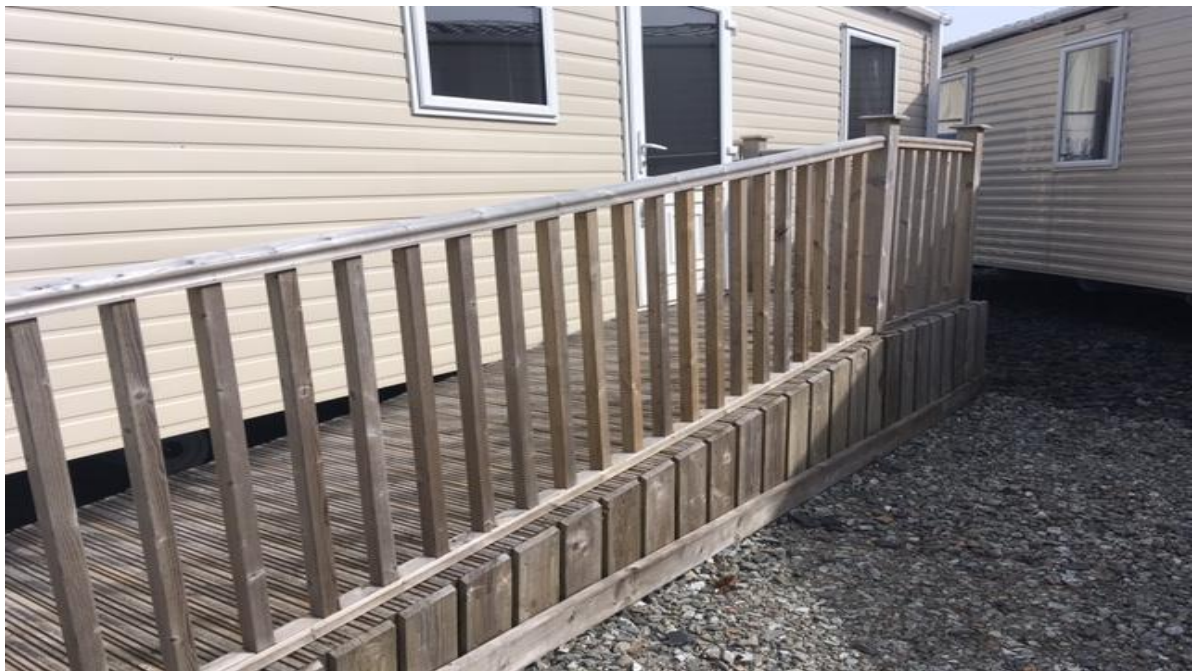
Miscellaneous Project Example 2 – Ramp to mobile home
